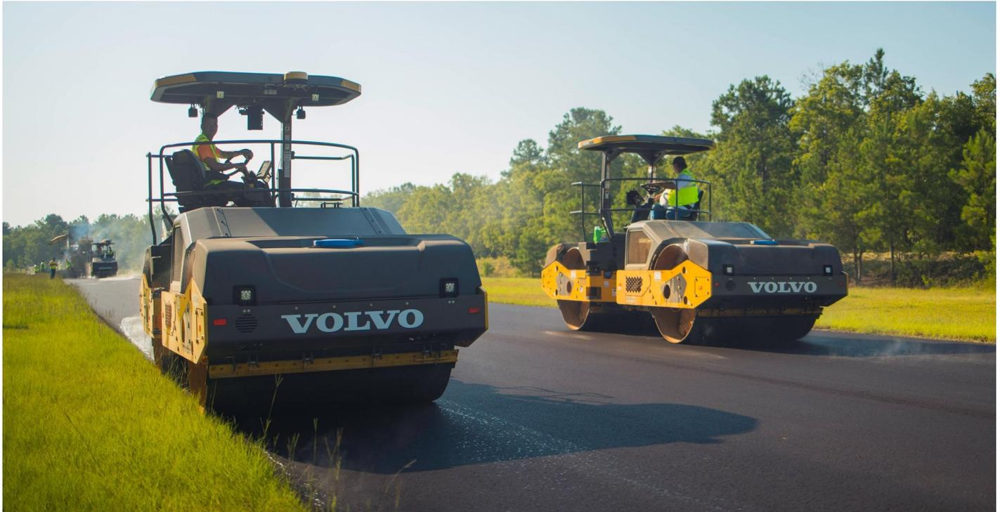
In addition, Lynch's River brought to the Carolina Motorsports Park project DD120 and DD110 rollers, noted for their advanced Intelligent Compaction systems that give an operator real time measurements of the asphalt temperature, the number of passes and monitor of the density of the mat itself.
